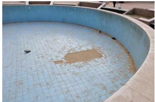
Central Fountain at Brotherhood Park before maintenance
